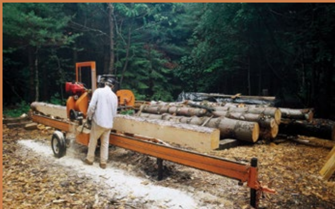
The timbers from the Unity site were sawed with a portable band-saw mill.
