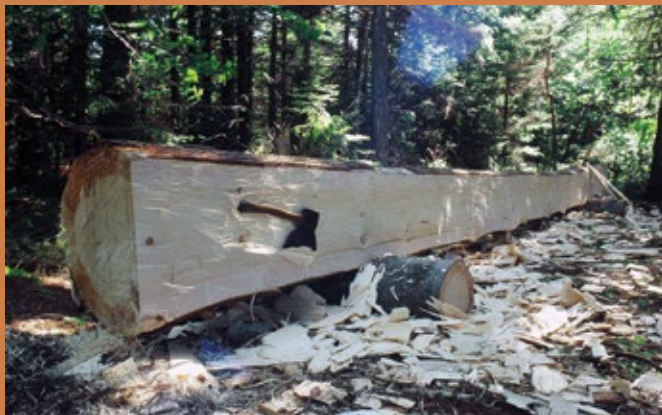
The two largest beams were hand hewn with a broad axe right in the forest.
