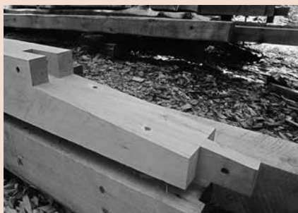
The 50 foot purlin plates and ridge beam are made of two shorter timbers "scarfed" together. This scarf utilizes two mortise and tenon joints and four pins.
